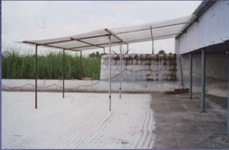
Drying Yard with Polycarbonate shed
