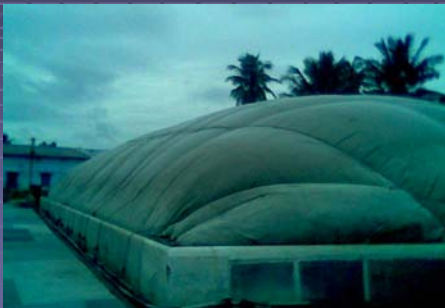
Effluent Treatment -Anaerobic Digester
